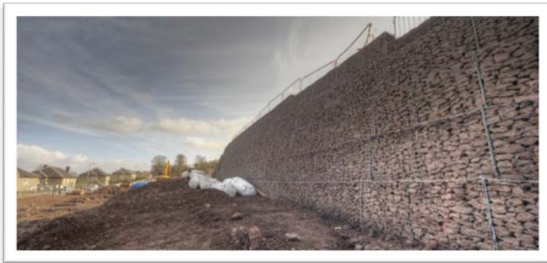
River Clyde Homes, Port Glasgow, Scotland
