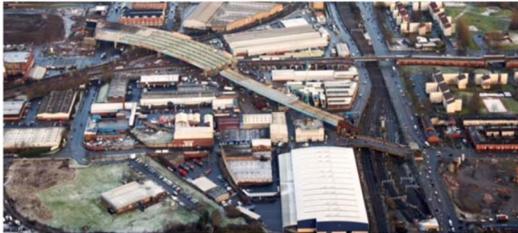
M74 completion, Glasgow
